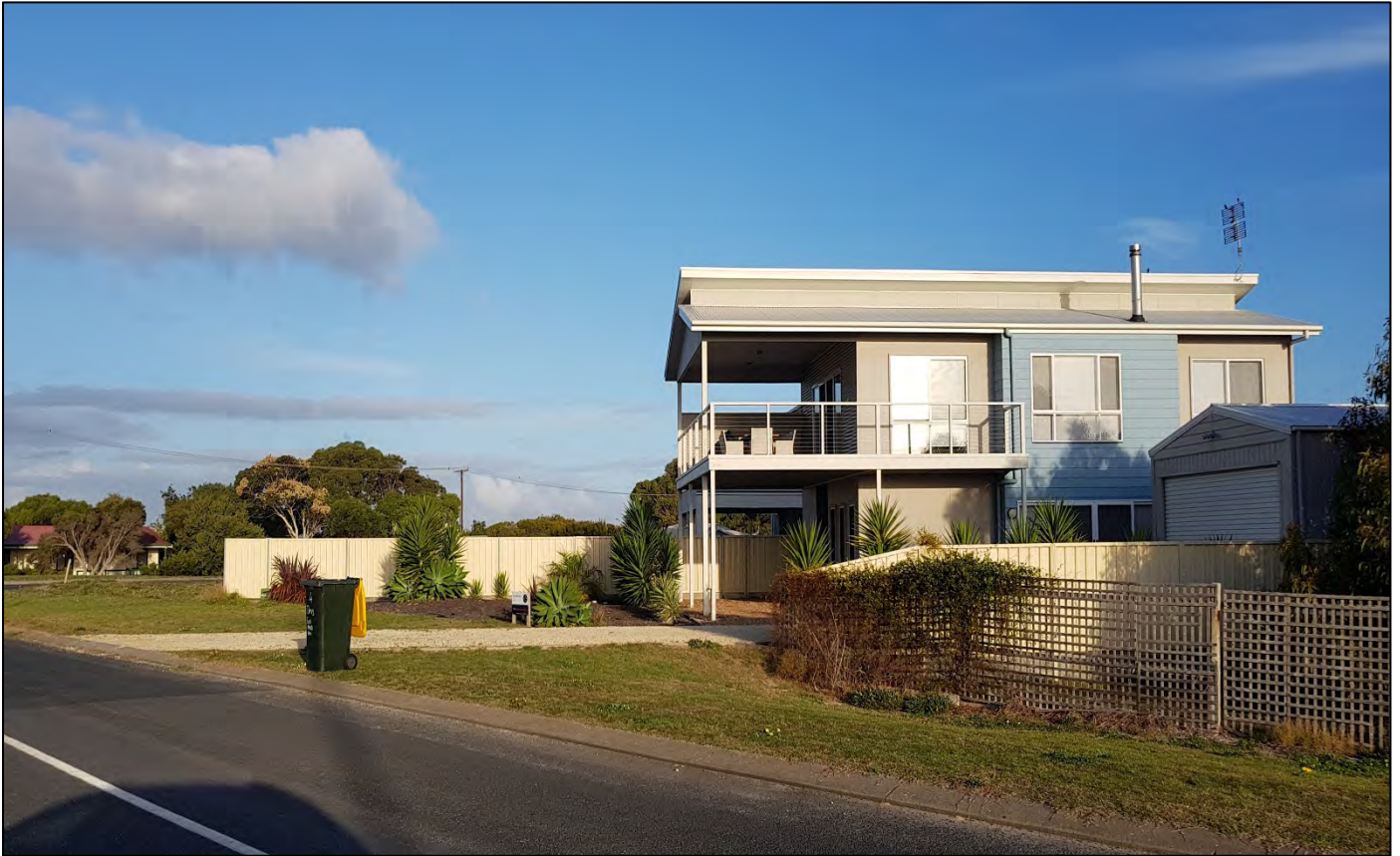
Figure 4: View south from Dennis Avenue toward the subject land (behind fence on the left-hand side) and two storey neighbouring property at 4 Dennis Avenue.
