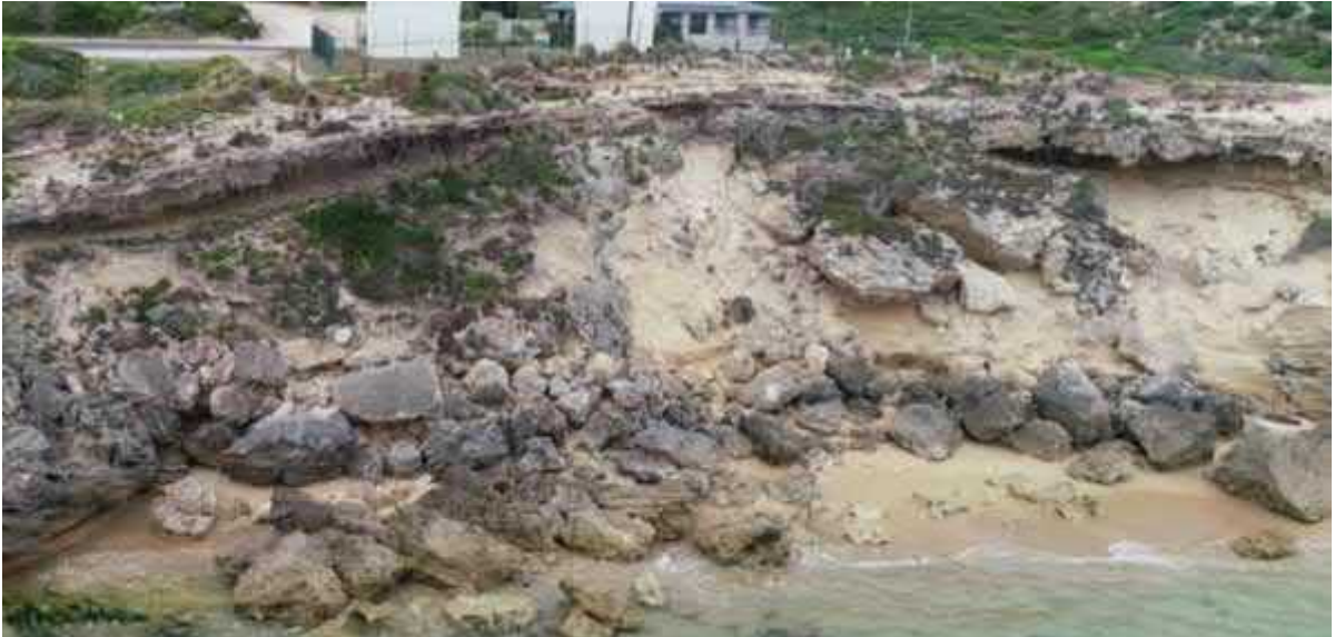
RZ14_0 - Undercutting of Cliff - Chainage 2150
