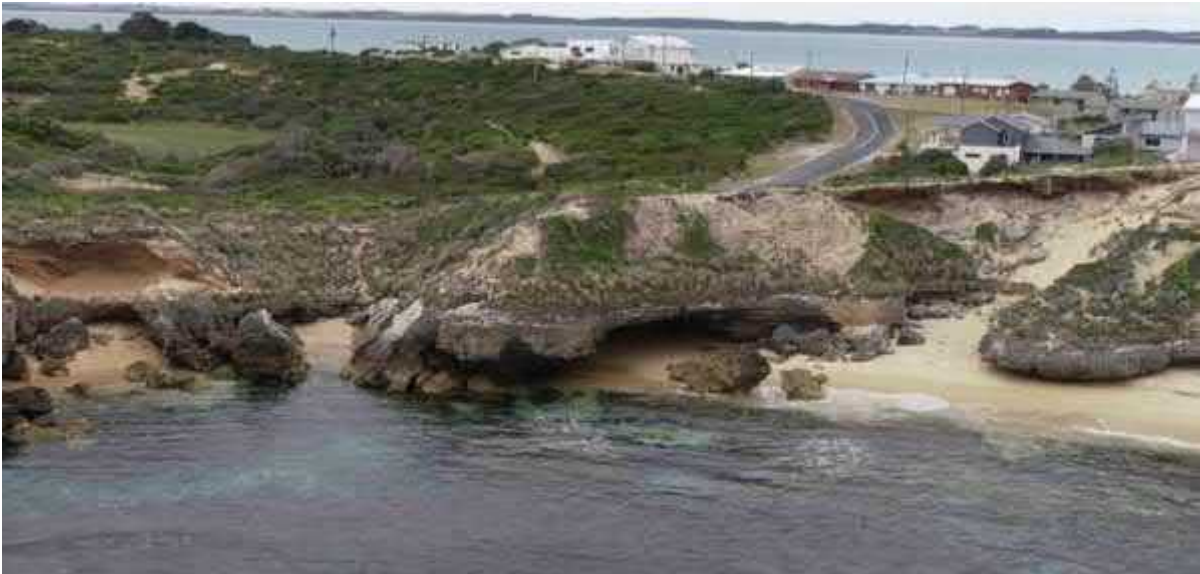
RZ13_0 - Overhanging of Cliff Face - Chainage 1900
