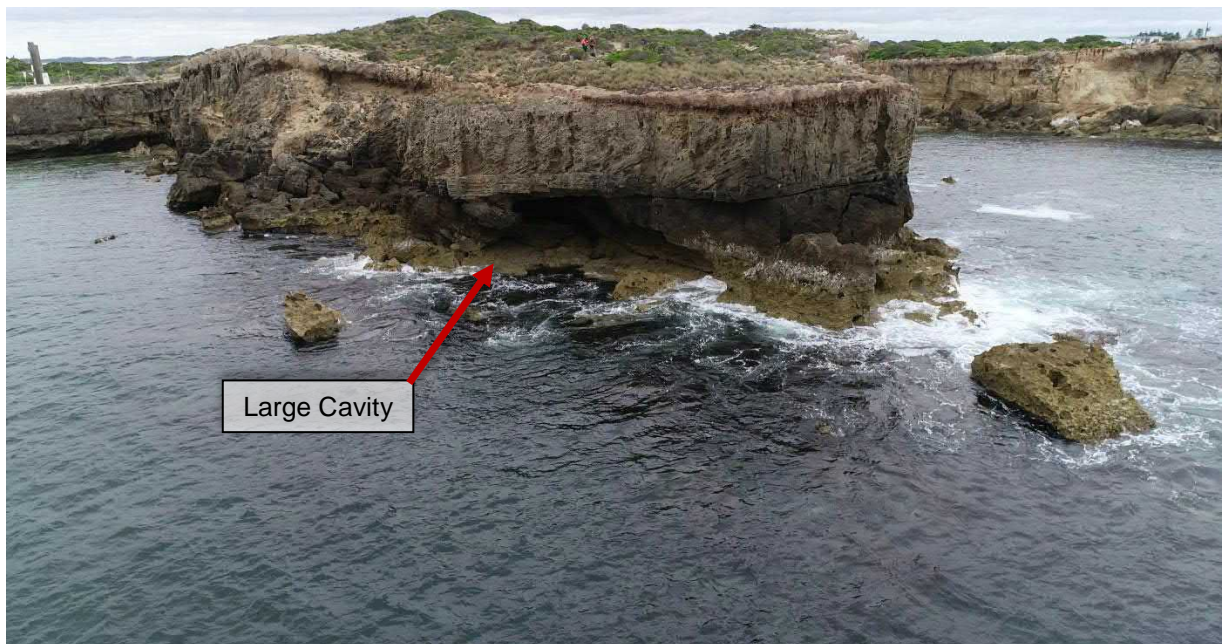
Figure 10 CH 825 – Large cavity under informal walking path.
