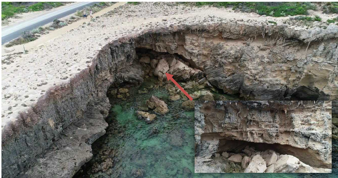
Figure 4 CH 690 to CH 720 - Obelisk Main Car Park Entrance – Undercut of Cliff Face
