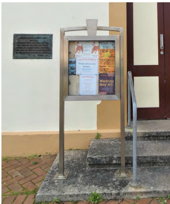
Above: The notice board at the main entrance to the Institute should be relocated.
