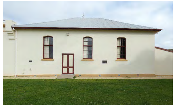
Above: North elevation of hall with a doorway that appears likely to have been a later addition.
