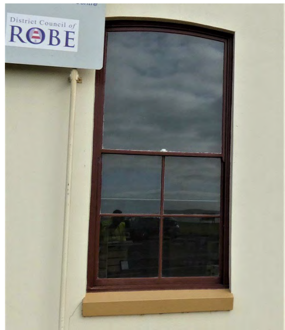
Above: Window to the north elevation of the library extension.
