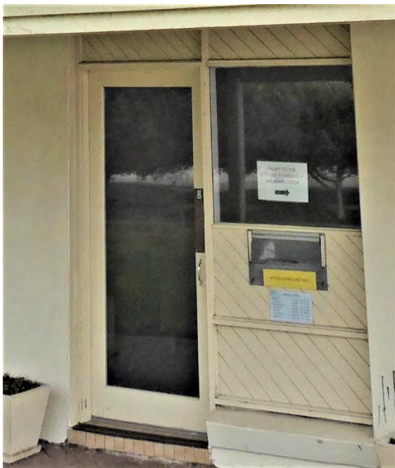
Above: Door and partially glazed side screen under the east verandah.
