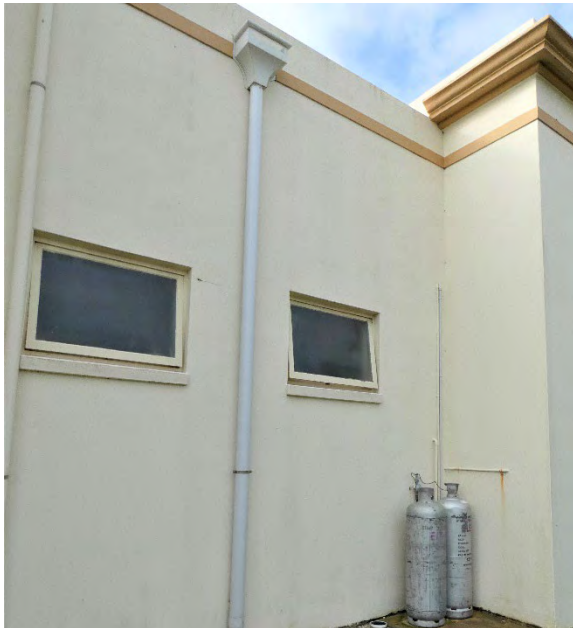
Above: Toilet windows along south elevation.
