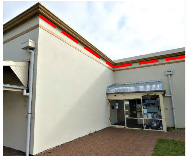
Above: View of corner entrance to the library and visitor centre. The dashed red lines show where the parapet box gutters run. Note the rainwater heads that the box gutters drain to.
