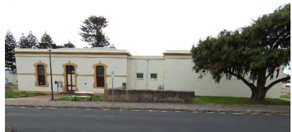
Above: Views of the roofs along the south elevation from the ground are difficult due to the parapets and low roof pitches.
