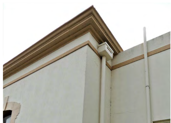
Above: Galv rainwater head at the east end of the roof of the original building along the south elevation.
