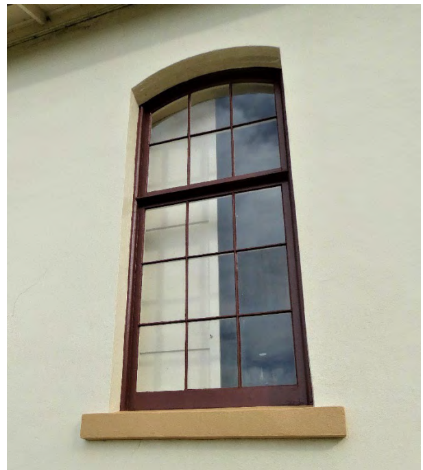
Above: Hall window along north elevation. Note the internal timber shutter.
