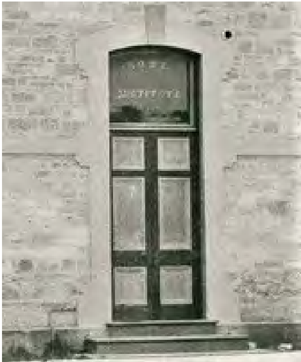
Above: Entrance door from photograph taken c. 1913. Note the painted lettering on the fanlight.
