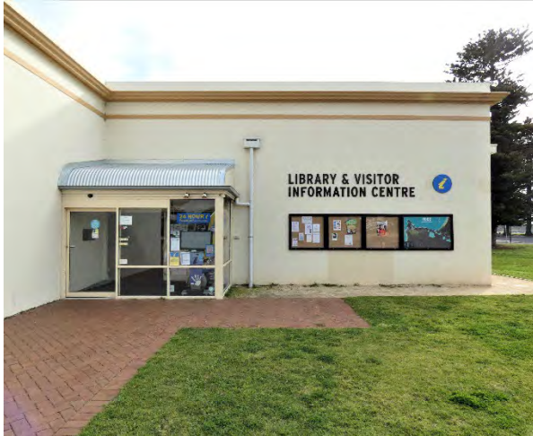
Above: Unattractive approach to the library and visitor centre entrance.
