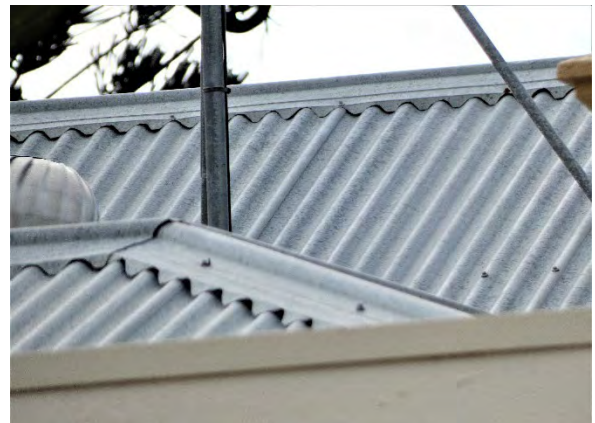
Above: In the foreground is the galv roof above the main entrance and side rooms. Beyond is the roof to the hall. Apart from some rusted roof screws the roof sheeting appears to be in good condition.
