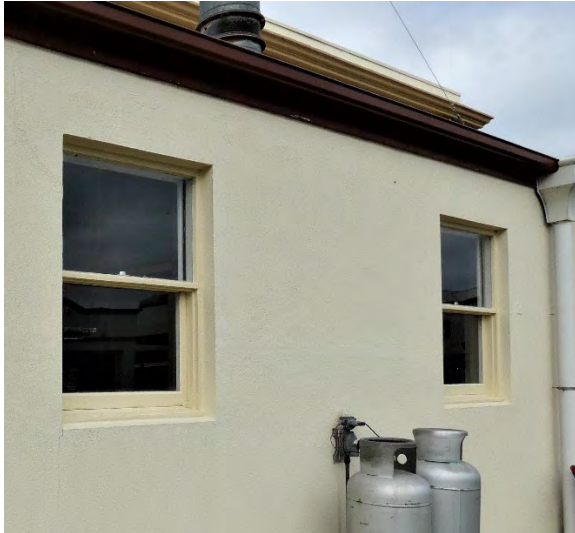
Above: Modern timber sash and case windows to the west extension.
