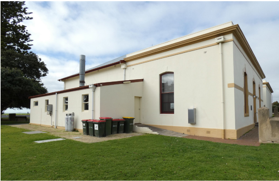
Existing west wall
