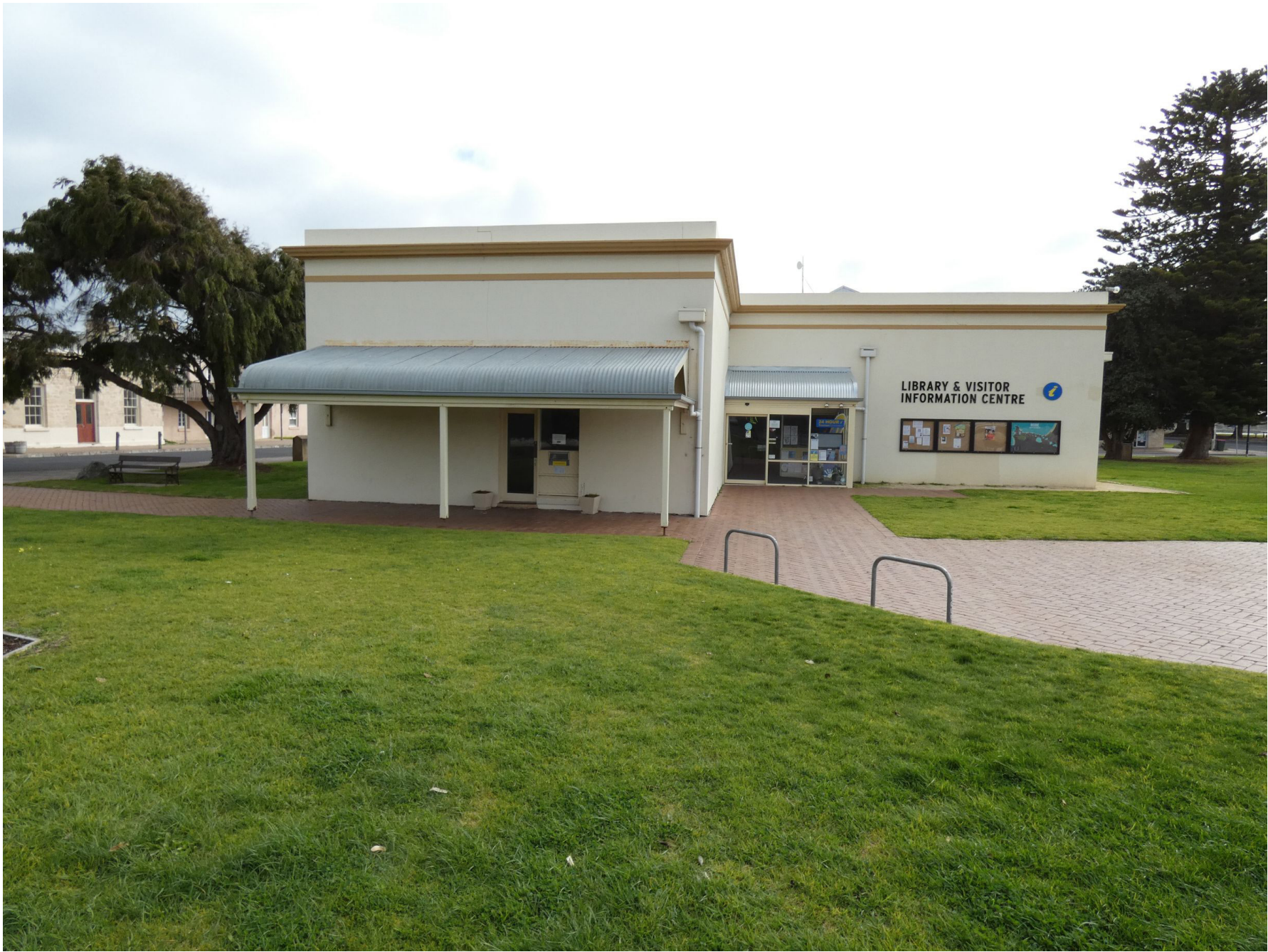
Existing east wall/main entrance
