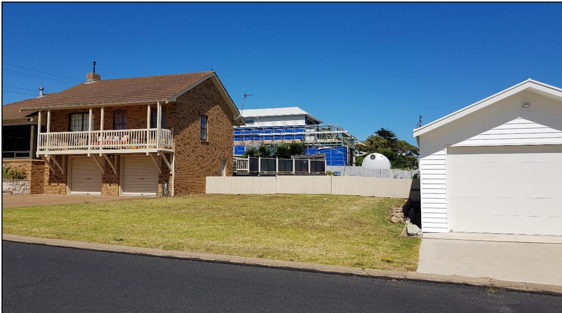
Figure 3: Subject land as viewed from Cooper Street showing the vacant portion of the land at the northern end of the allotment
