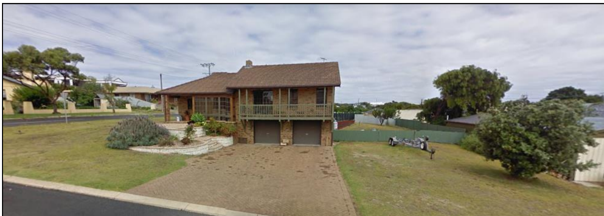
Figure 1: Subject land from Cooper Street
