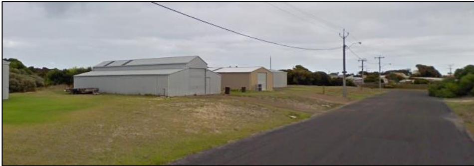
Photo 4 – sealed & un-kerbed industrial road at Southend.
