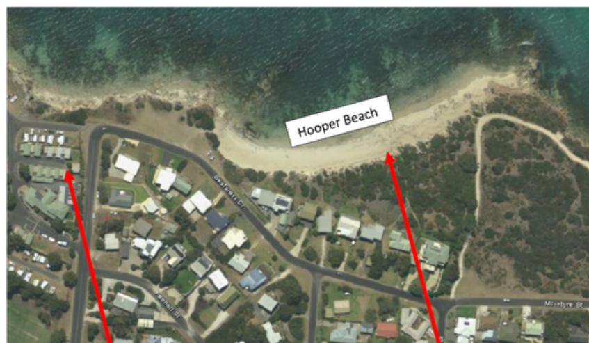
Location of existing navigation beacon
