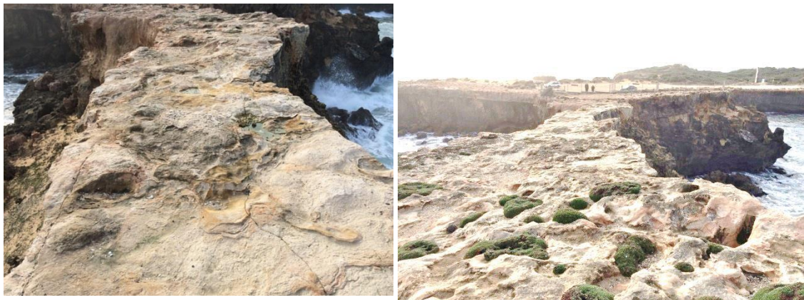
Photo 4: Access to the Obelisk is via a narrow uneven landmass. Note the cracks in the surface rock.
