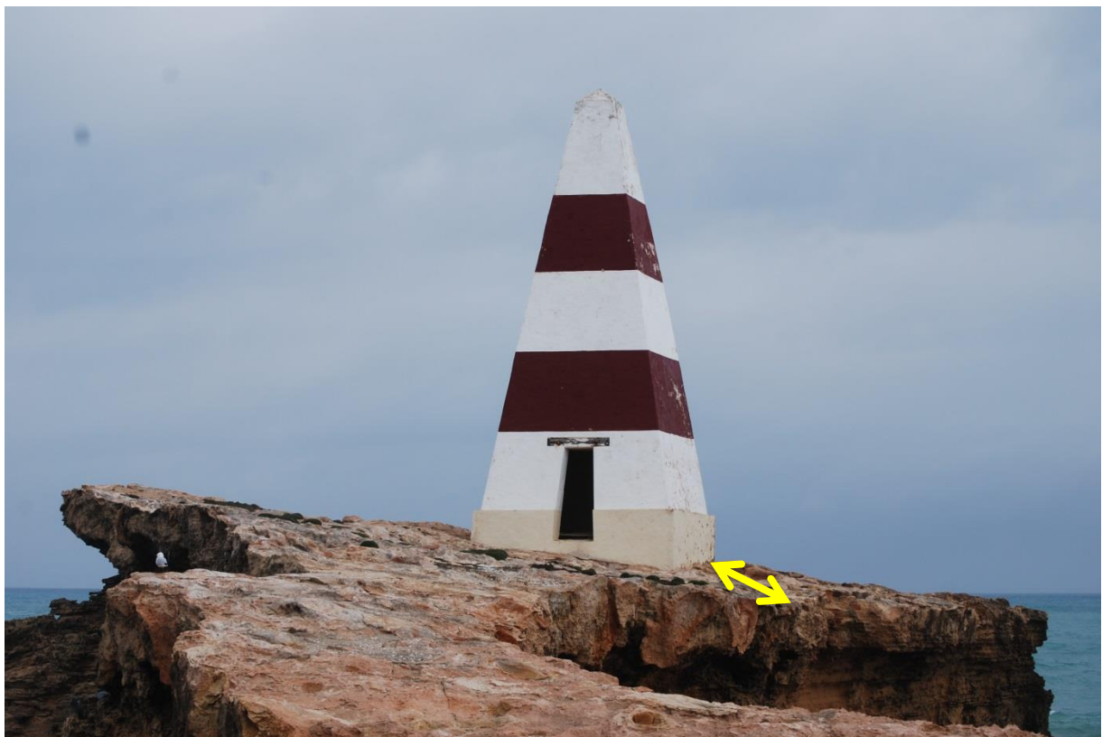
Photo 2: View looking West. Note width of north eastern footing of the Obelisk is approximately 3.8m. (yellow arrow denotes distance). Also the ledge is undercut by atleast 0.5m.
